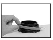
3. Ensuring the fitting with gasket are flat against the spa wall and centered within the hole, add the Load Washer ring to the back so the cone locates into the hole.
