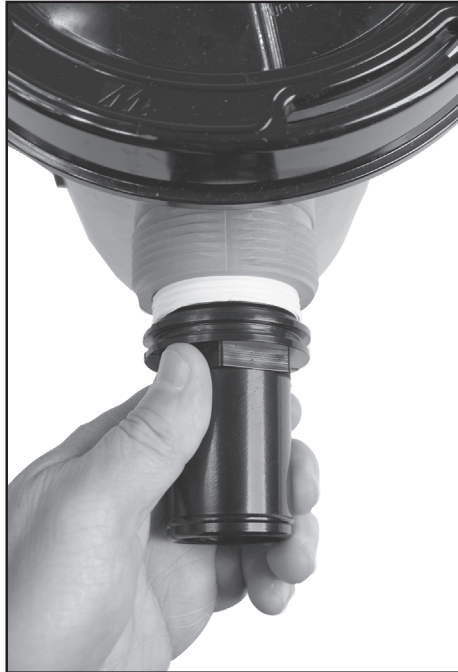
2. Thread onto pump trap inlet.
