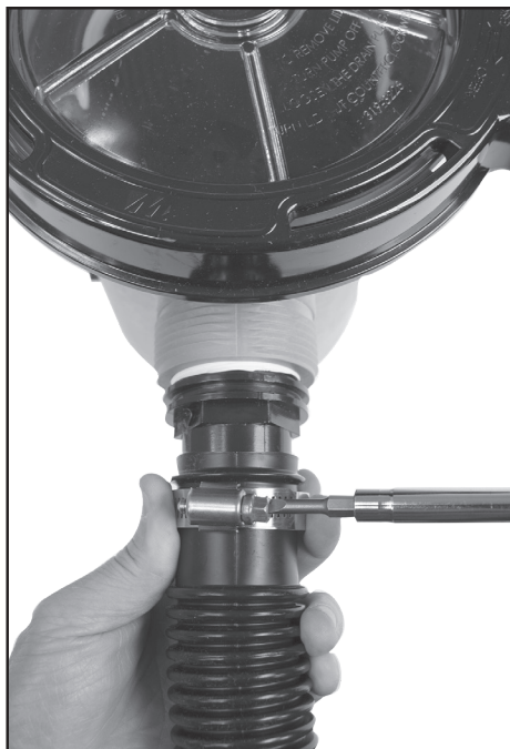
5. Using hose clamps provided, install hose on hose adaptors on the pump trap inlet...
