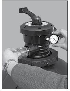
8. Install waste adapter (clear fitting) into waste port. Apply Teflon tape to PSI gauge threads (4 wraps) and thread into multi-port valve.
