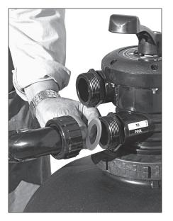
Put 1 ½" gasket into return sweep assembly and install onto pool outlet port. DO NOT OVER TIGHTEN.
