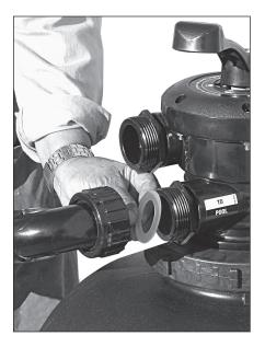
8. Put 1 ½" gasket into return sweep assembly and install onto pool outlet port.
