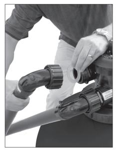
9. Take pump to filter hose assembly and put 1 ½" gasket into nut on smaller end with sweep 90°. Thread onto pump outlet port.
