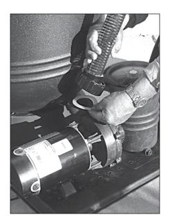
10. Put 2" gasket into nut on hose labeled "TO VALVE PUMP PORT."DO NOT OVER TIGHTEN.
