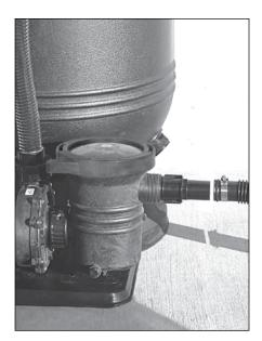
13. Install 6 ft. corrugated hoses by loosening hose clamps and sliding over hose ends. Install hose onto pump basket hose fitting by pushing on and tightening clamp. Install other end of hose onto skimmer and tighten clamp.
