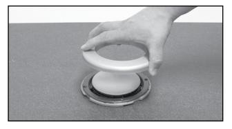
6. Position the trim ring over the wall fitting and speaker body. Rotate clockwise until the trim ring locks into place, securing the speaker.
