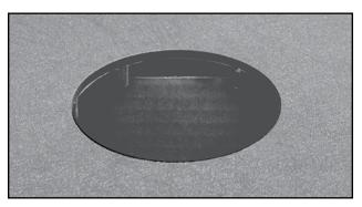
1. Locate an area on the spa wall that has a flat surface at least 6  $\frac{1}{2}$ " in diameter. Drill a 4 7/8" diameter hole through the spa wall.
