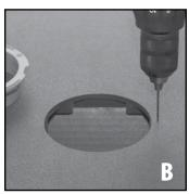
3. Using the speaker wall fitting as a template, (A) drill four 5/64" diameter holes around the perimeter for the four #6 x 1" oval Phillips-head screws (B).
