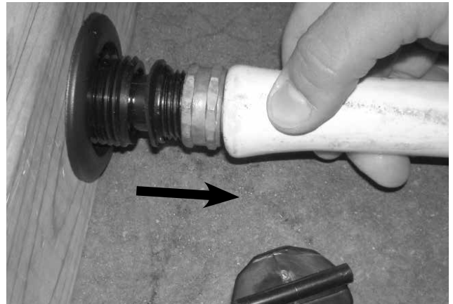
8. Pull the hose outward to allow water to flow. Push inward to shut water flow off.
