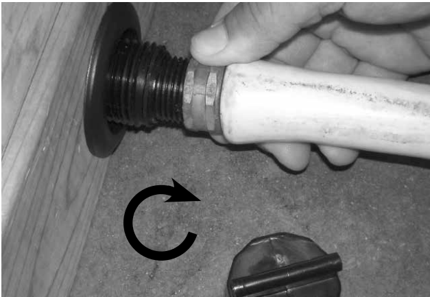
7. Thread hose onto the spa drain.
